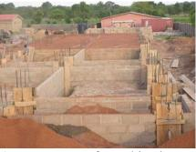
As you can see from this picture lots of construction is going on at Bethany village. We have dug a foundation of 5 ft. Presently, the whole foundation is finished up flow level.
